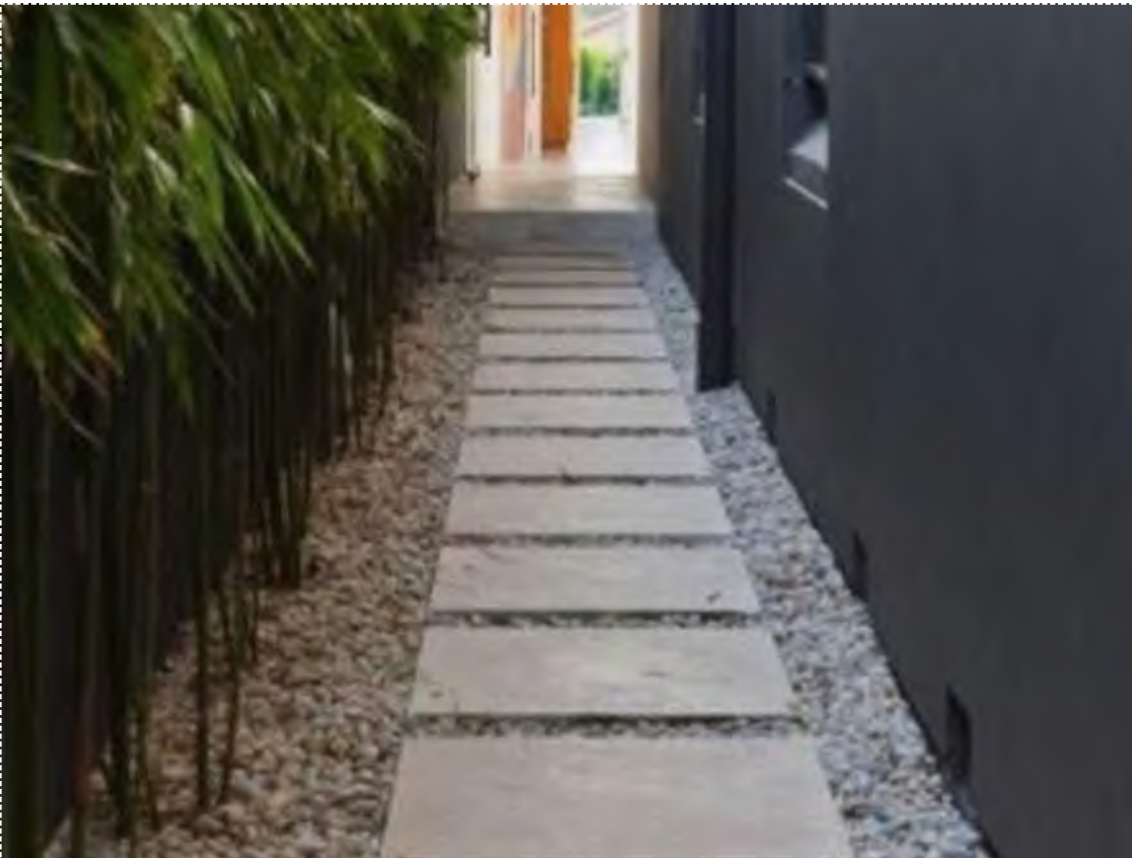
Concrete stepping stones in gravel / pebble mulch to side lot area
