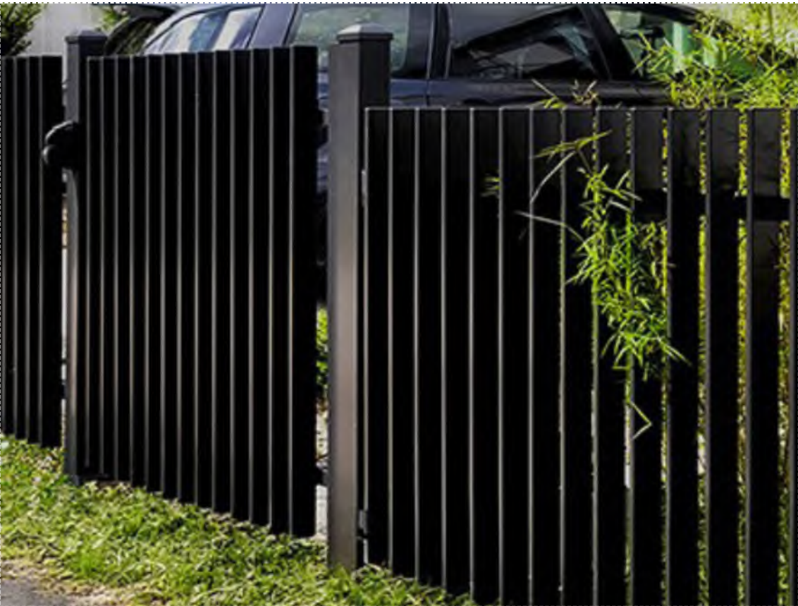
Blade fencing and gate
